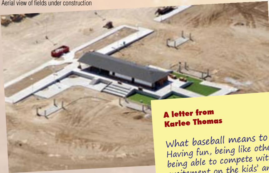
Aerial view of fields under construction
